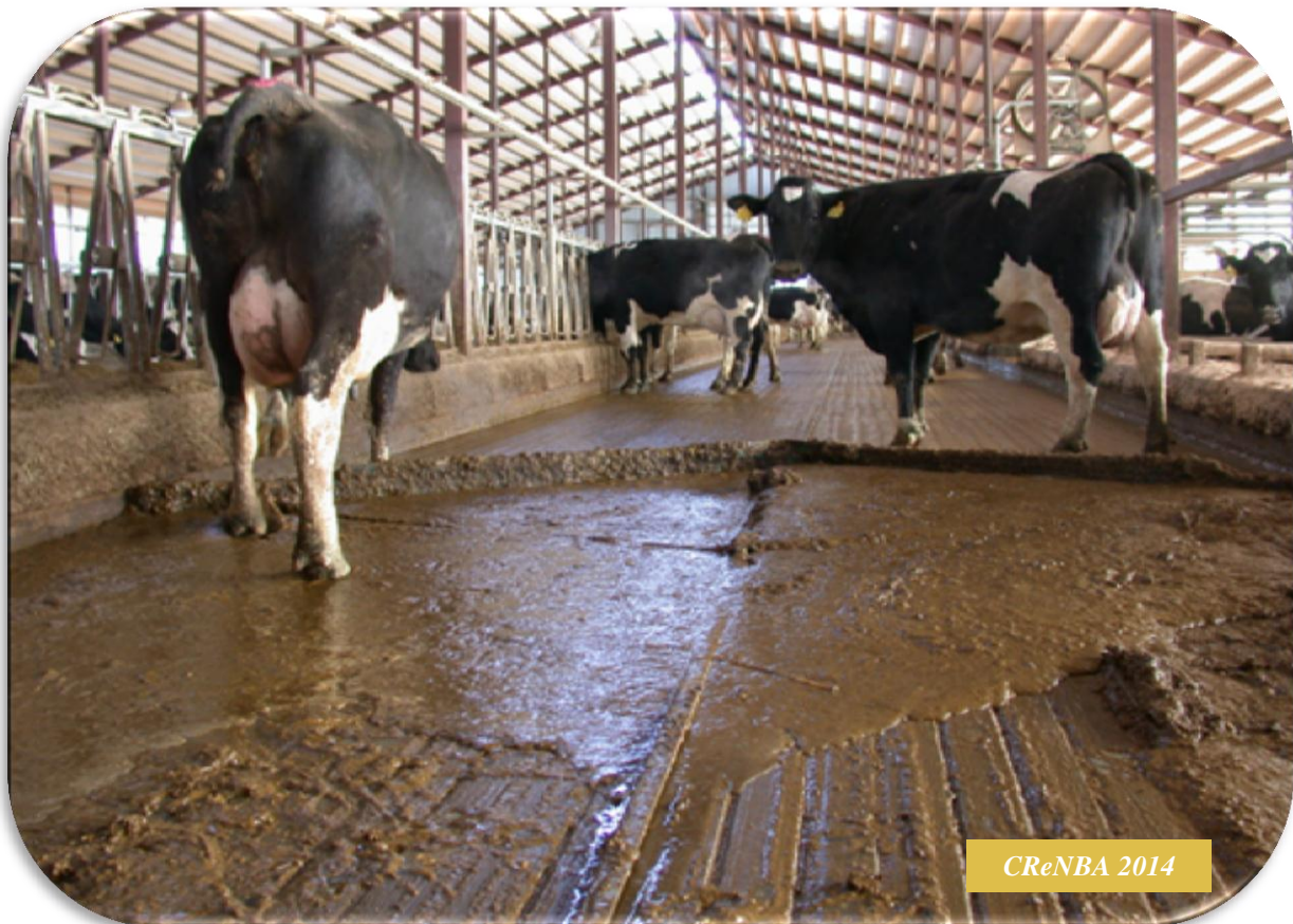
Figure 20 - Example of grooved concrete flooring which allows animals to move about without slipping.
