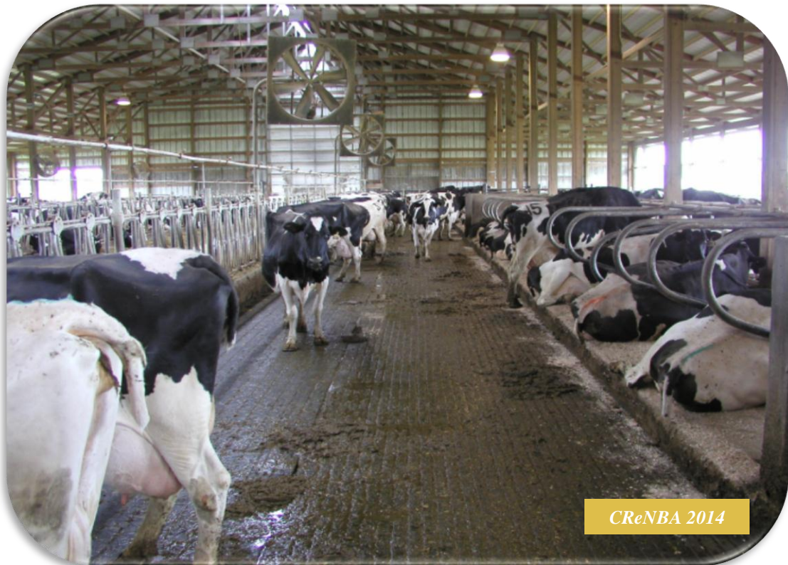
Figure 6 – Example of a clean and dry environment.
